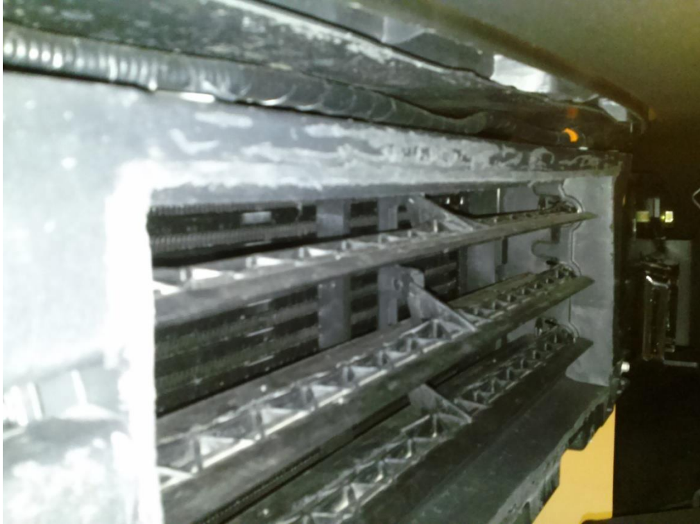
Figure 4 (Louver w/ shroud cut away at base)
