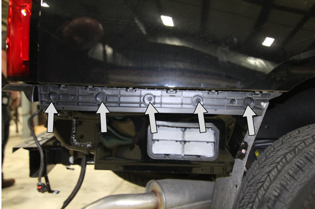
Figure 6 - CLIPPING BRACKET REMOVAL – VIEW FROM BELOW
