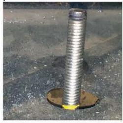
Screw the all thread into the upper bracket and push it through the pre-drilled hole. Mark the all thread just above the top of the frame.
