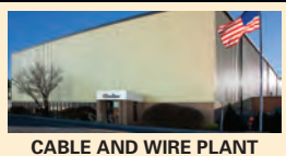
CABLE AND WIRE PLANT
