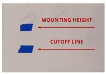
12. Mark the mounting height on the wall or garage door using tape.
