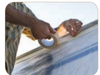
Mask off sidewalls to protect graphics.
