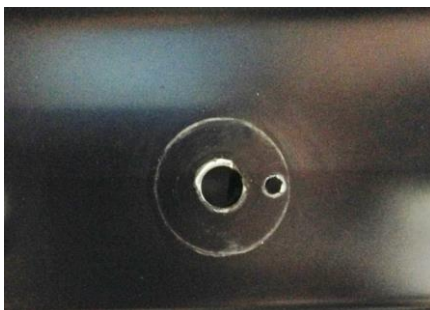
Figure 10 - Drill Anti-Rotation Hole
