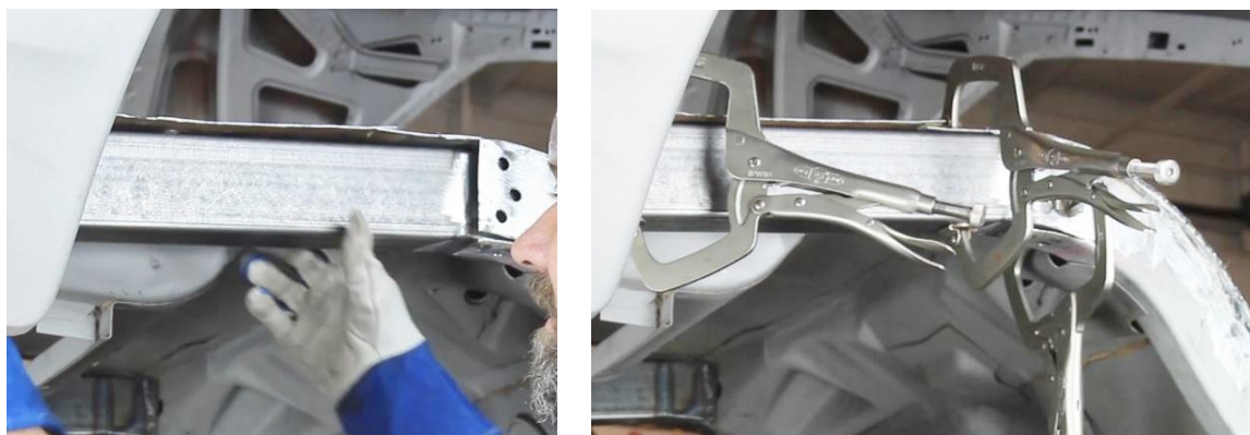
Figure 21 – Clamp Detroit Speed Frame Rail in Place
