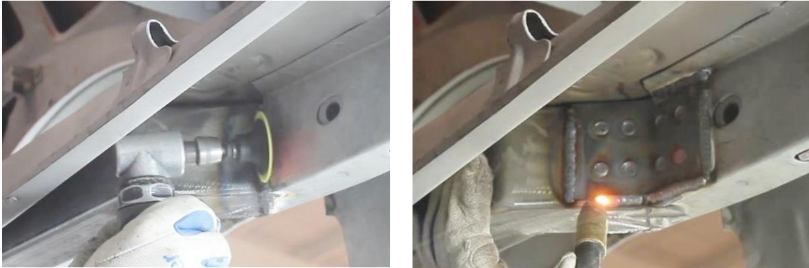
Figure 23 - Weld Inside Frame Rail Doubler Plate
