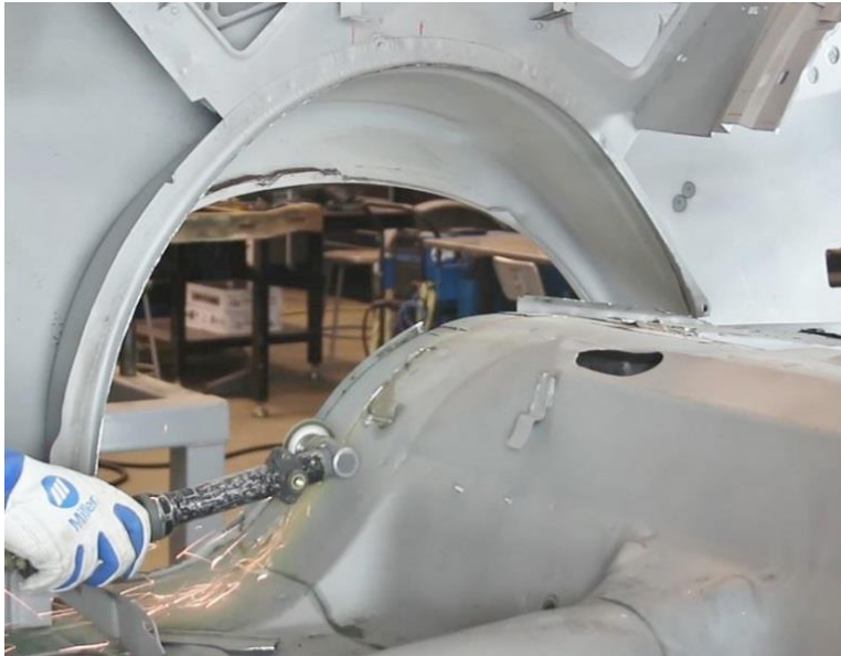
Figure 9 – Remove Floor Pan Section
