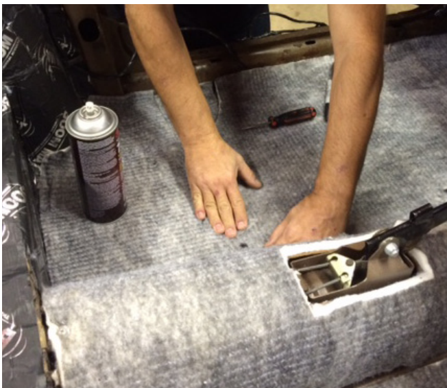
UC Lite trimmed and peeled back awaiting spray adhesive.
