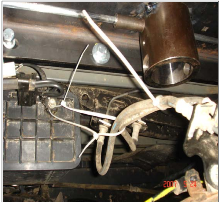
MODIFIED BRAKE LINES USING CABLE TIES
