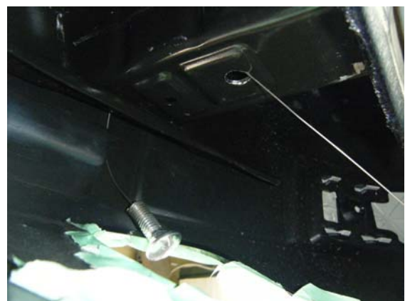
DRIVER SIDE FISHWIRE LOCATION
