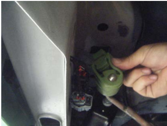
EXHAUST HANGER REMOVAL
