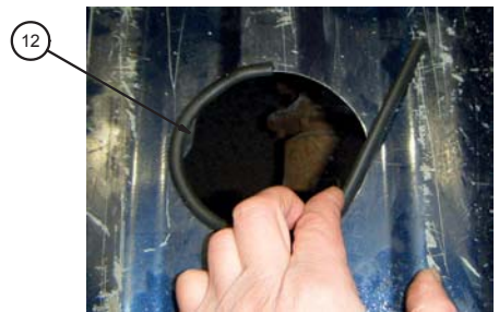
U-EDGING INSTALLED AROUND EDGE OF 4" HOLE IN TRUCK BED
