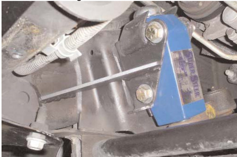
FIGURE C - Gusset welded in center of brace; SS175 installed.
