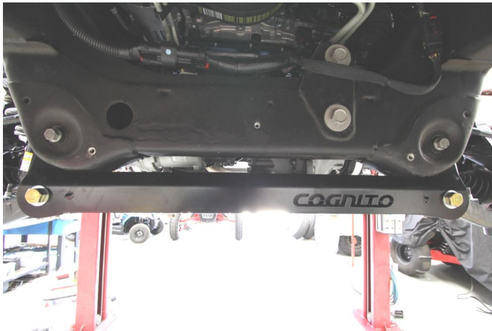
Figure 14: installing front crossmember
