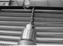
STEP 6 Drill 1/8" holes at each marked location.
