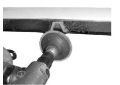
STEP 4 Using a sander or sanding block sand all rough edges smooth. Repaint if neccessary.
