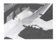
STEP 5 Set the grille in place in the opening and scribe around the vertical posts where they contact the frame.
