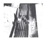
STEP 7 Set the grille inserts in place for positioning. The ends of the bottom grille have a shallower angle than those of the top grille. Clamp the insert and mark the location of the vertical bars on the inside lip of the opening.
