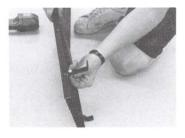
STEP 6 Install the L-shaped mounting brackets supplied on the bottom side of the tabs on the top of the grille. The leg of the L should point up. Tighten them finger tight.
