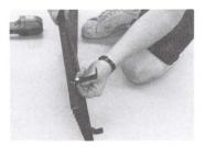
STEP 6 Install the L-shaped mounting brackets supplied on the bottom side of the tabs on the top of the grille. The leg of the L should point up. Tighten them finger tight.
