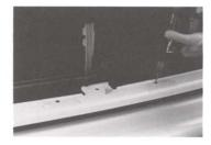
STEP 3 Remove the grille and drill the four 1/4" holes in the bottom panel.
