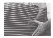
STEP 2 A Position the new grille in the opening, then tip the top outward in order to reach behind it and mark the mounting hole location.
