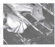
STEP 11 With a rotary tool (or rattail file), grind notches into the horizontal bars for the vertical supports.
