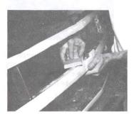
STEP 8 With 80 grit sandpaper, smooth and round the edges where the "egg crate" was cut out. Follow up with 150 grit paper to smooth the surface and remove the old finish in preparation for painting.
