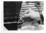
STEP 7 With the grille in desired position, mark each point where the round vertical bars contact the grille frame on top and bottom.
