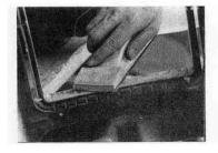
STEP 4 Sand the surface with sandpaper on a block to prepare it for painting.
