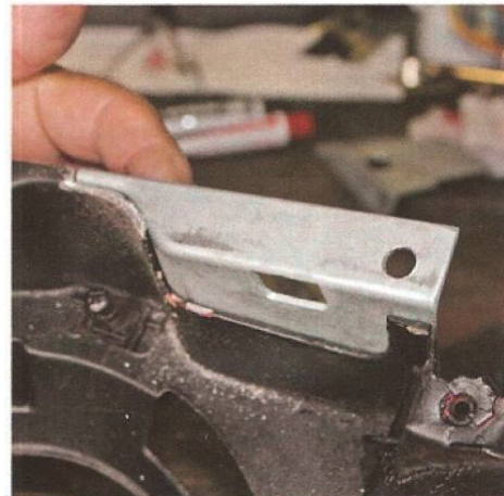
3 After dressing the edges with a file, the repair patch can be positioned on the bucket for a test fit. Make sure all casting flash and burrs are removed.
