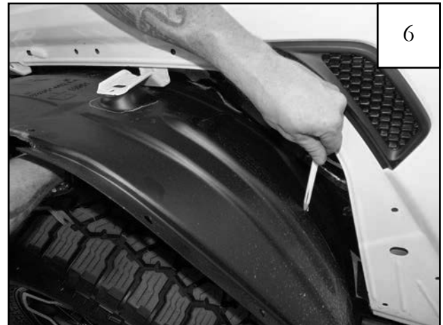
Using sheet metal as a guide, mark the rear portion of the splash shield with a grease pencil in preparation for trimming. The splash shield should be flush with the sheet metal after being trimmed. NOTE: If trimmed too little, flare won't fit; if trimmed too much, shield won't stay behind flare. Rear portion beneath vent may be left long.
