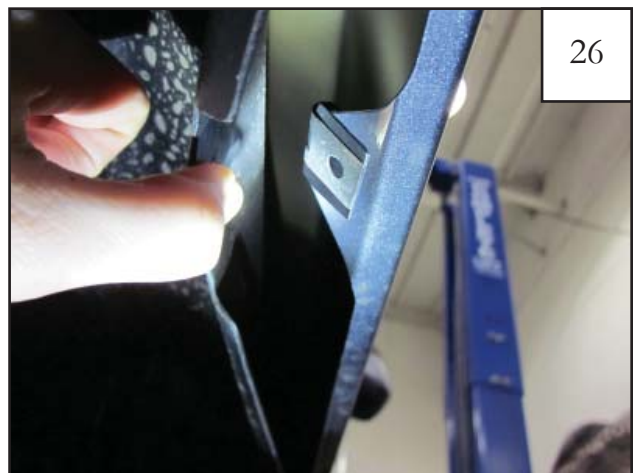
Slide Clip (CL1-0022) over factory hole locations behind wheel well liner over tab installed in previous step. Two locations. Reference Step 22 for locations.
