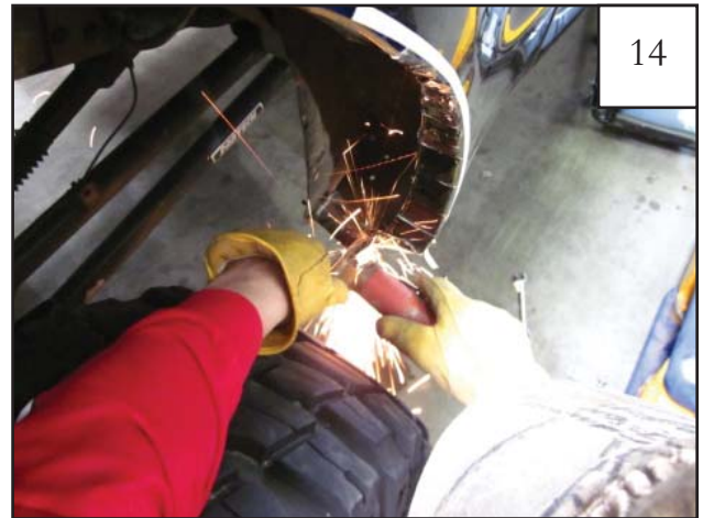
Using cut-off wheel, cut marked lines along bottom flange.
