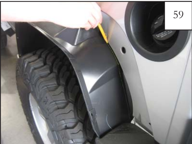
Using sheet metal as a guide, mark the splash shield with a grease pencil in preparation for trimming. The splash shield should be flush with the sheet metal after being trimmed. NOTE: If trimmed too little, flare won't fit; if trimmed too much, shield won't stay behind flare.
