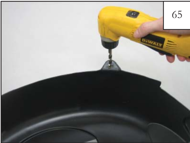
Use a drill and 5/16" drill bit to drill through mark made on rear mounting tab.
