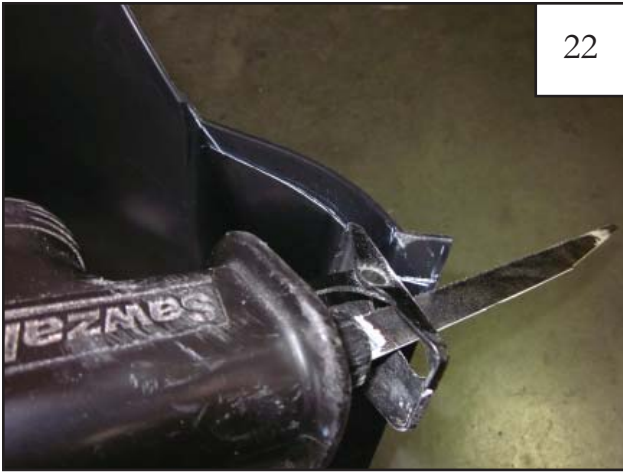
Using a sawsall, cut of section marked in step 21.
