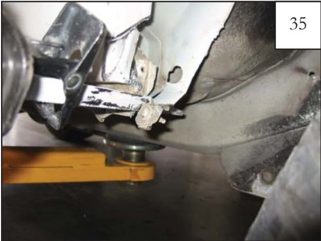
Use a saw to cut off remaining sheet metal and bolt.
