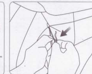
③ Connect the monitor power extending line to the reverse light power line, anode to anode, cathode to cathode, then fix the cables with the rubberized fabric.
