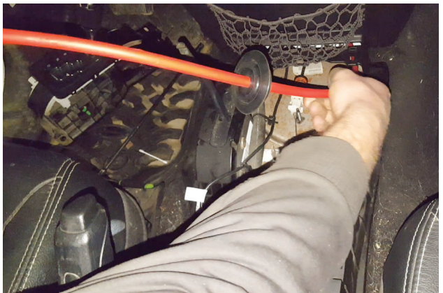
17. Route threaded end of cable down through entry point in cab out to bottom side of vehicle.
