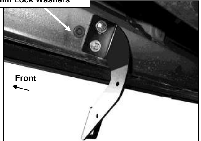
(Fig 7) Passenger side center Bracket installation
