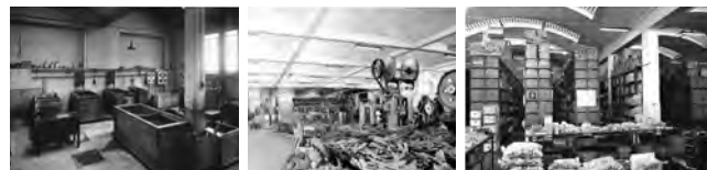
1950 Galvanising department 1955 Shearing department 1960 Shipping warehouse
