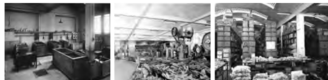
1950 Galvanising department 1955 Shearing department 1960 Shipping warehouse
