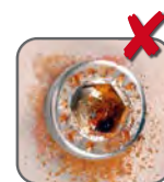
STAINLESS STEEL + NO STAINLESS STEEL = RUST
