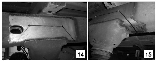
**4e)** Connect the lines marked for the inner and outer templates across the bottom of the frame.(**Photo 15**)
