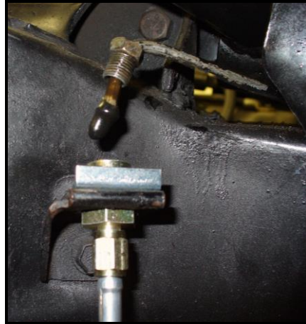
Figure 1: Vinyl cap installed onto hardline
