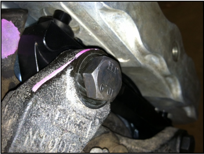
Figure 7: Bracket correctly installed (view from inboard side) Note: No washers are needed below bolt head
