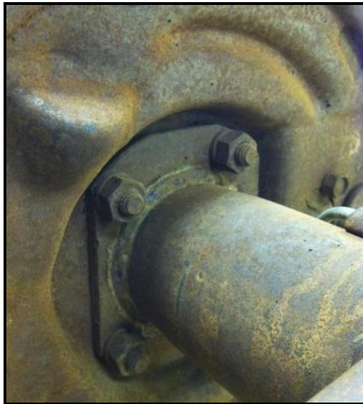
Photo shown of OE fasteners and OE backing plate (Driver's side)
