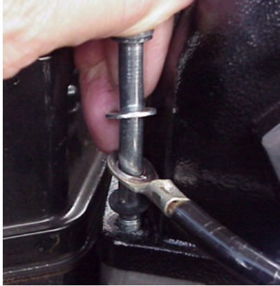
Figure 3 - Installing Ground Wire, Note Rubber Washer Below Ring Terminal
