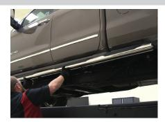
Attach the side bar to the brackets with six of the 10mm hex bolts, locking washers and flat washers.
