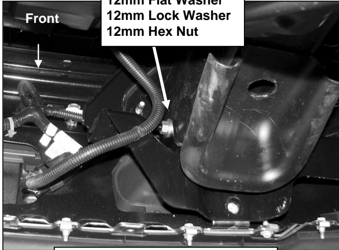
(Fig 8B) Passenger side Frame Bracket installation pictured
