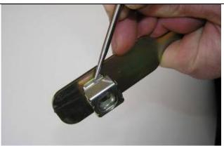
10. Fit an M12 cage nut to each of the captive nut plates 3193741.
