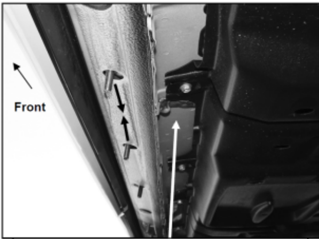
from all locations before installing Brackets
