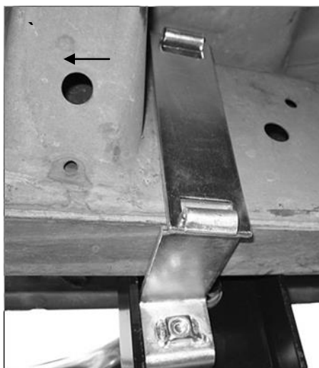
(Fig 5) 99-03 Rear Bracket Connector Installation Pictured
