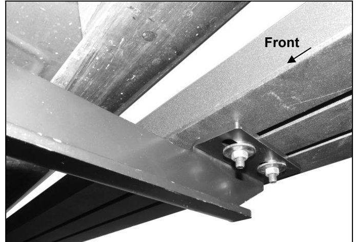
(Fig 17) Passenger/right center side complete install
