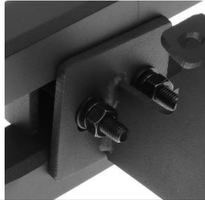
(Fig 7) Driver/Left side bracket installed
