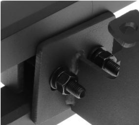
(Fig 18) Driver/Left side bracket installed
